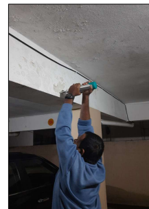
Rebound Hammer test
